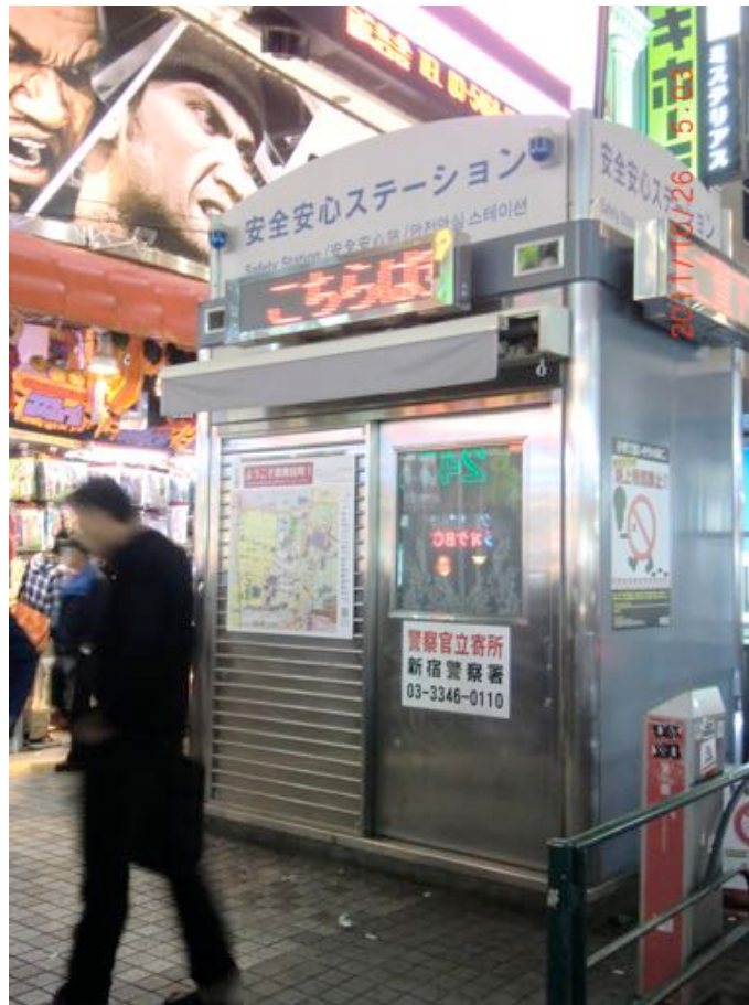
Figure 3. The pre-fabricated police station in Kabukicho
