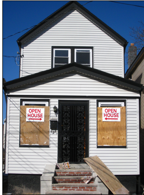
Figure 4: Foreclosed single-family home in Queens, NY, 2011 (photo credit: author’s own)
