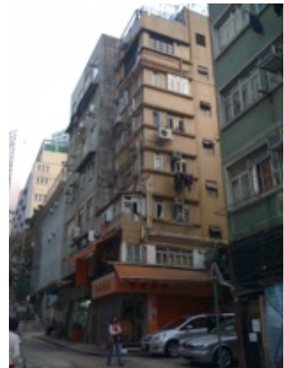
Top: Chi Residence ’s latest project in Wan Chai in partner ship with the property owner. The bottom two: Serviced Suite hidden in tenement apartment in Sheung Wan.
