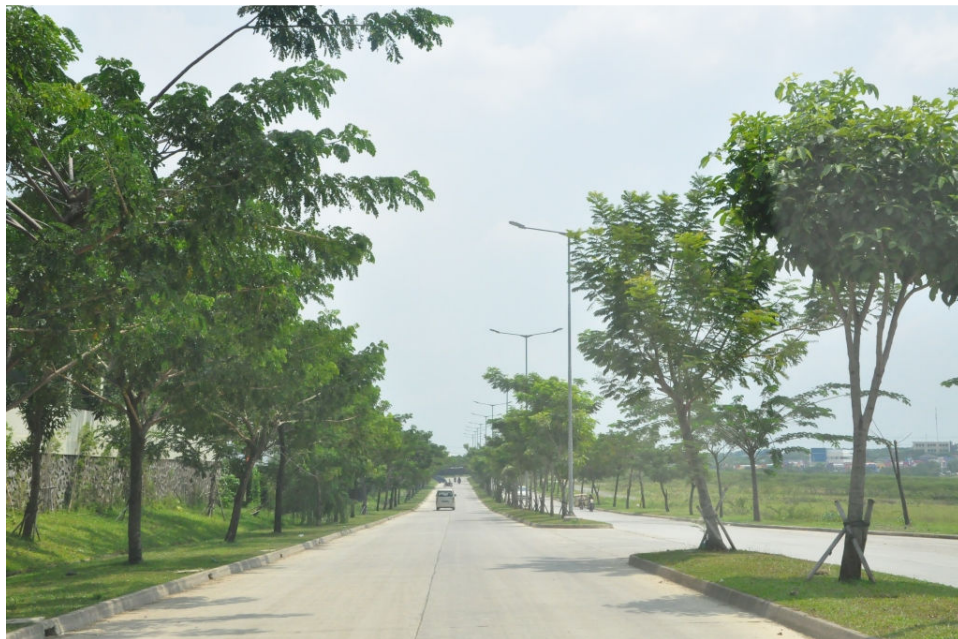
Figure 4 A connecting road built through public-private partnership in Cikarang
