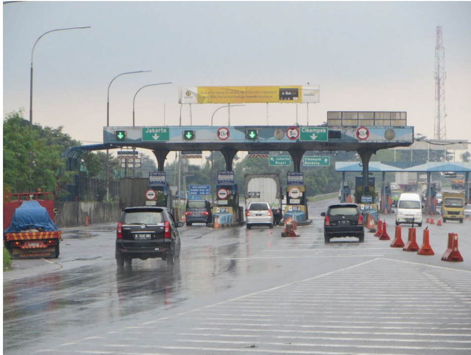
Figure 3 A toll road interchange built by a private industrial developer in Cikarang
