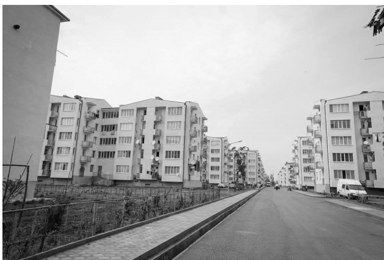
Figure 4. The residential buildings in the new district in Poti, Western Georgia. Source: MRA, 2015.
